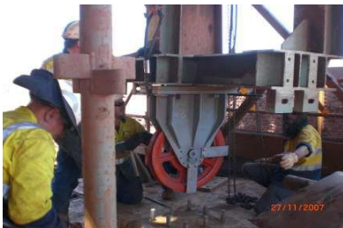
Paraburdoo Train Load-out Conveyor 25 (CV25) – New Hybrid Take-up System. Designed, Procured and Implemented During a Three Days Maintenance Shut Down at Paraburdoo Mine in 2007 in Western Australia.
